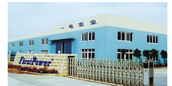
FirstPower Yixing Plant
